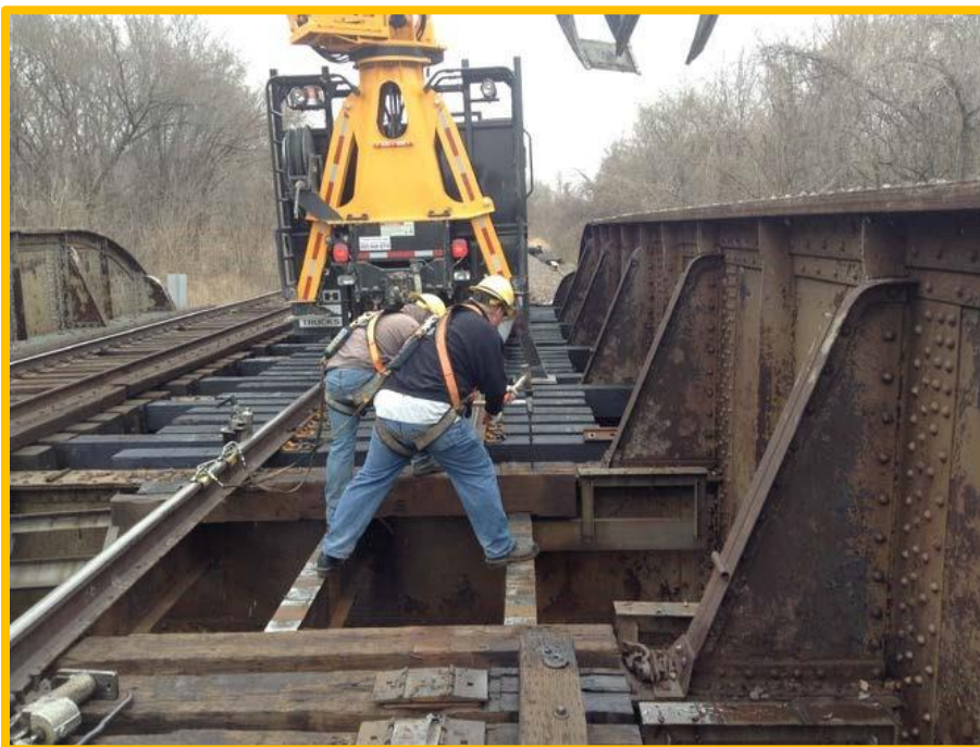
BMWED B&B workers working on a through-plate girder bridge, date unknown.
